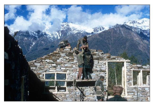
**Figure 5.** Laborers construct the main living quarters for Cronin and McNeely's staff (photograph by J. McNeely).
