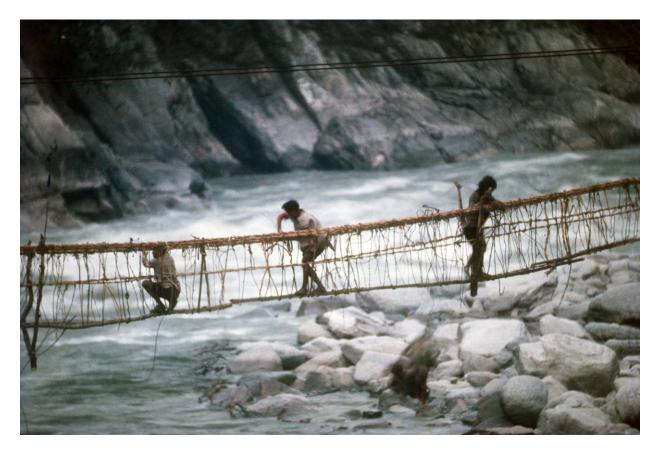
**Figure 3.** The bridge made of woven vines over the Arun below Num, being repaired and upgraded by porters prior to its crossing by more than 285 porters, each carrying an 80-pound (36 kg) load (photograph by J. McNeely).
