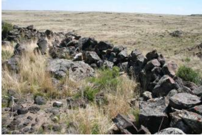
Figure 5. Substantial rock structure from INL (Hellofasite).
